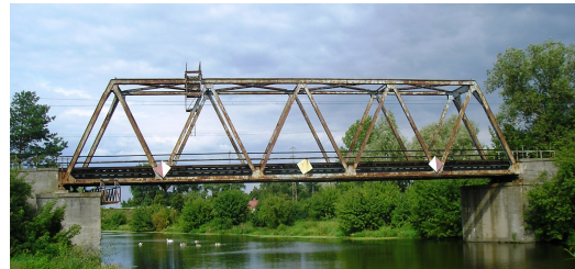
Fig. 1 Railway truss bridge monitored in Nieporet
